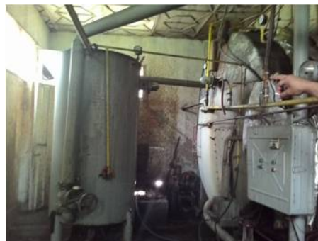
Photo 2. Still operating pilot biogas plant No. 2 in Tokmok, Chui Oblast
