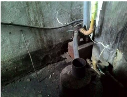
Photo 1. Inside of operation room of the pilot biogas plant No. 4 in Chon Kyzyl-Suu village, Issyk-Kul Oblast. It shows poor condition of facilities like heating stove, pipes which were seriously damaged last winter when water got inside the room and got frozen as it can be seen from the line on the wall.
