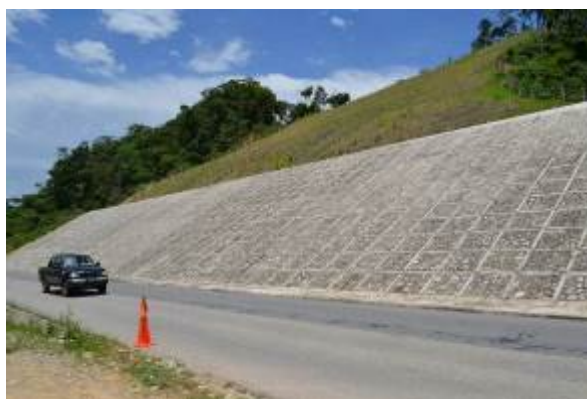
Slope Protection Works on National Road 1 in Variante, Tarija Department (Pilot Project)
