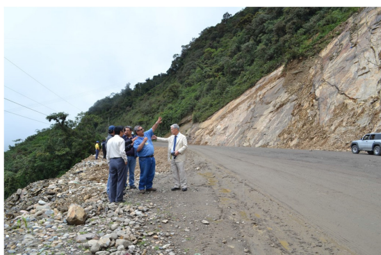
Site of slope failure on National Road 4 Due to the extensive slope failure, the road width is much larger than usual.
