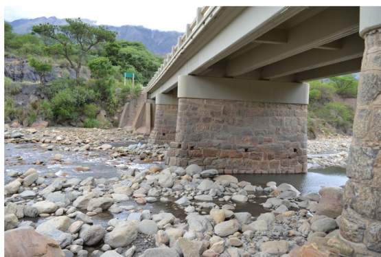
Repair of Popo Bridge on National Road 7 Cracks in the main girders and floor plates were repaired, giving the bridge the strength to withstand the weight of large vehicles. (Pilot project)
