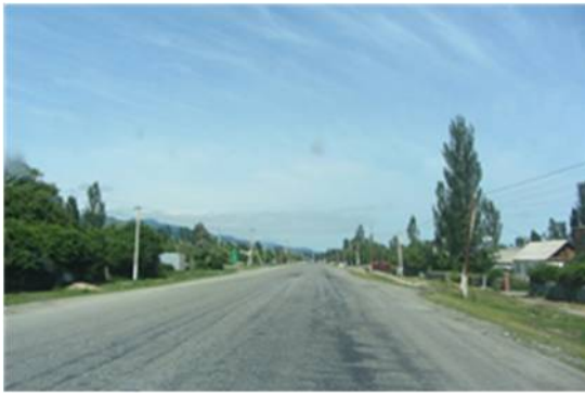
(Issyk-Kul Road after the pothole patchwork)
