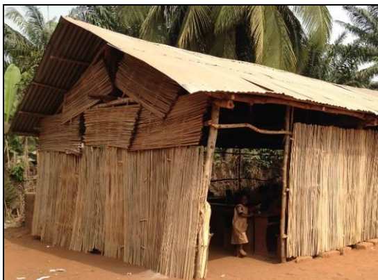
Photo (Left) Simple classroom
