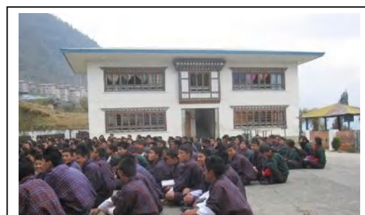
Four-classroom building Chukha School, Chukha District
