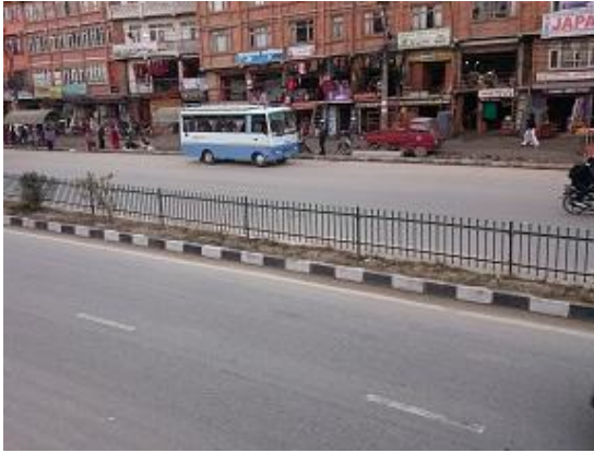
Picture 1 Guard fences at the median strip
