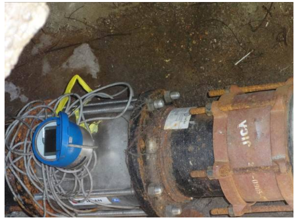
Macrometer provided by the Project for ANDA Metropolitan Region which is still in use and functioning.
