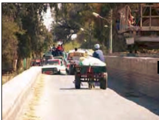
Photo 3: Regulator Bridge and Road prior to Rehabilitation (narrow with a 4m width and prominent congestion)
