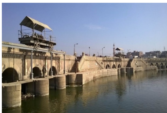
Photo 5: Dairut Regulator Group (The mobile pulley above opens and closes the gates. The structure is generally old.) (At the time of the ex-post evaluation)
