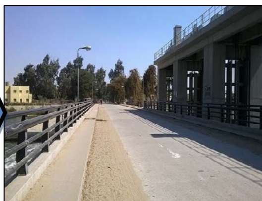
Photo 4: Regulator Bridge and Road after the Rehabilitation (expanded to 10m wide by this project)
