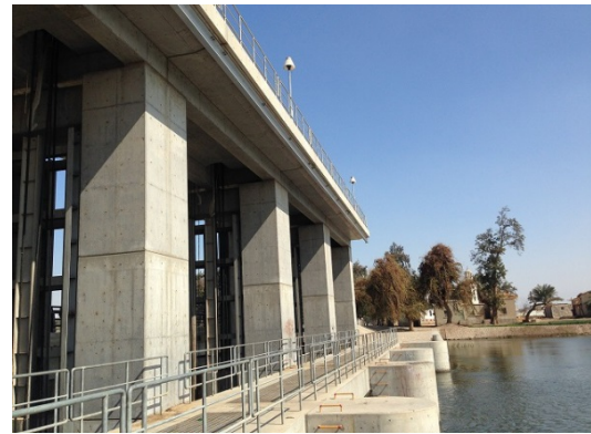
Rehabilitated Dahab Regulator
