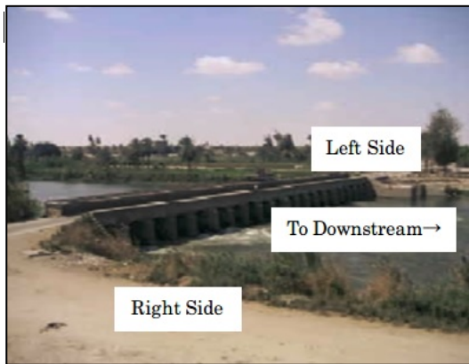
Photo 1: Dahab Regulator before rehabilitation
