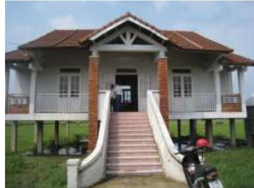
Evacuation center constructed through this project (An Xuan Village in Hue Province)
