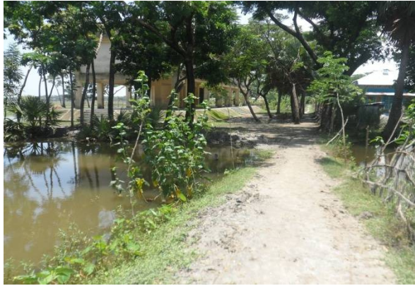
General condition Entrance cyclone shelters
