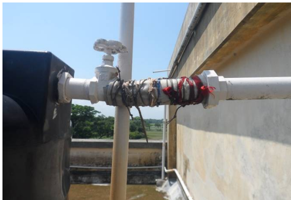
Damaged rain water cistern system.
