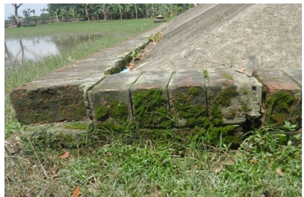
Guide wall and slope from the Dias.
