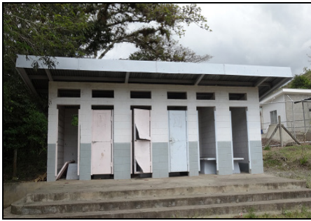
External view of pit latrines (six booths. Doors have come off in three of them and cannot be used)
