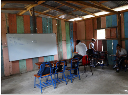
Classroom before improvement:
