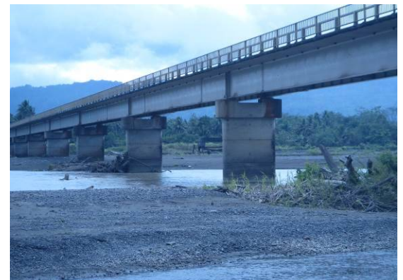
Bride Piers of Markham Bridge
