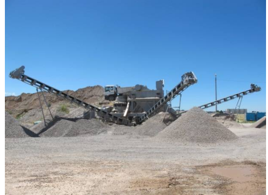
(Aggregate Plant constructed in Chui oblast.)
