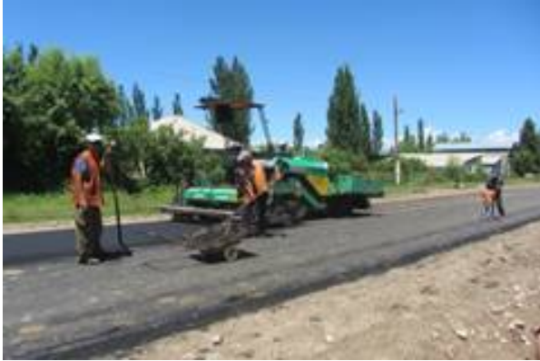
(Road being rehabilitated with asphalt in Issyk-Kul Oblast)
