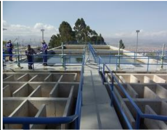
Aranjuez Water Treatment Plant
