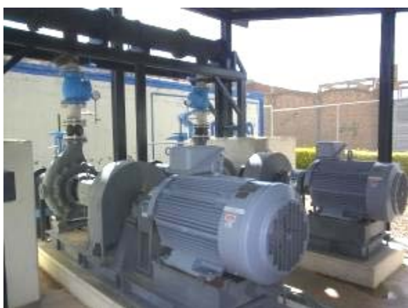
Siglo XX Pumping Station
