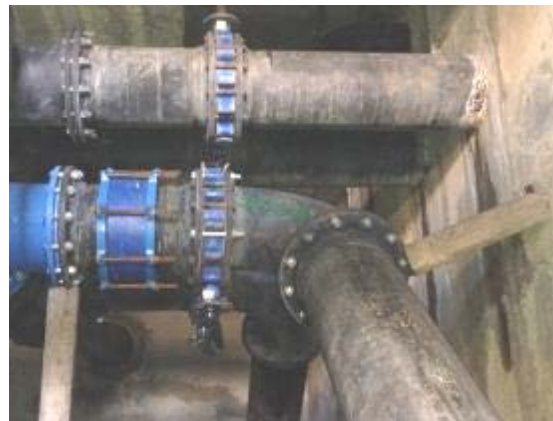
The pipe repaired at the Aranjuez WTP
