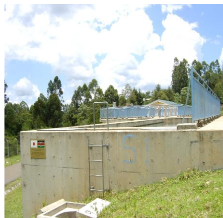
Sedimentation Pond of the Water Treatment Plant
