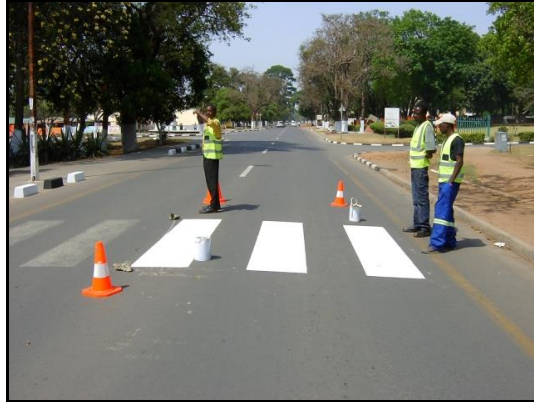
Maintenance work on the markings on Independence Way, Ndola
