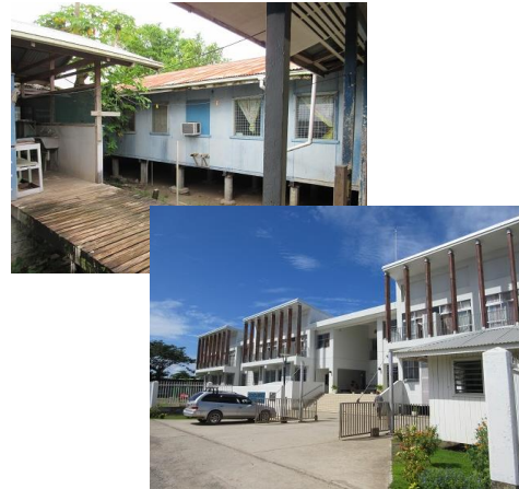
Old and New Gizo Hospital Buildings
