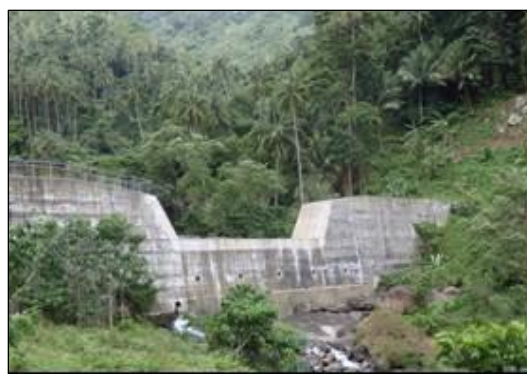
Sabo Dam (Upper Dam)
