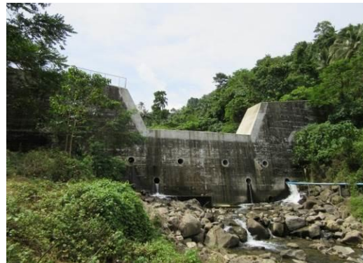
Sabo Dam (Lower Dam)
