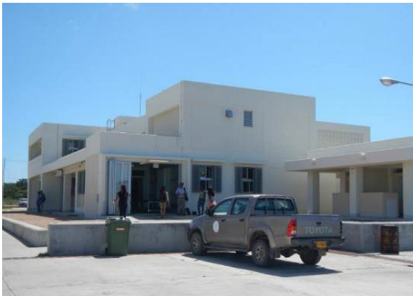
Entrance to the fish handling room of the fisheries facilities (at the time of the ex-post evaluation)
