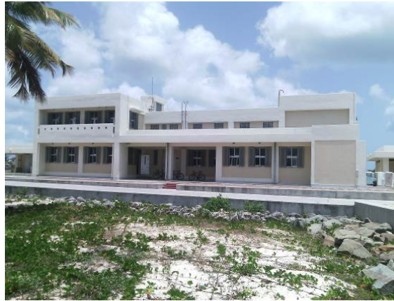
The Fisheries Complex constructed under the Project in Barbuda Island Codrington area
