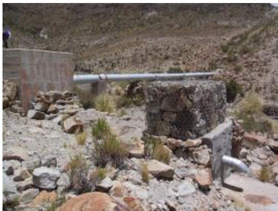
The dirt removal facility
