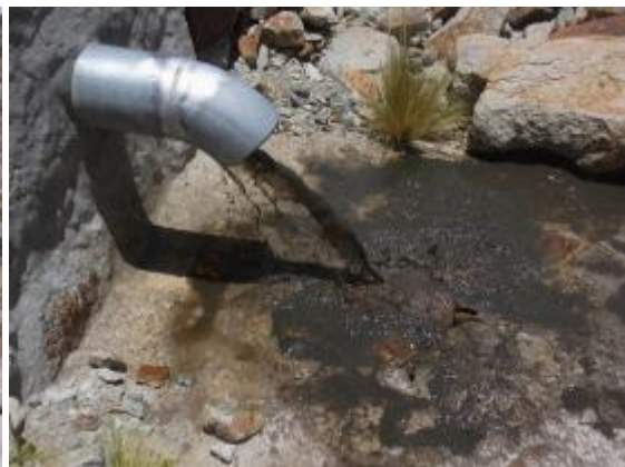
Operation of the dirt removal facility
