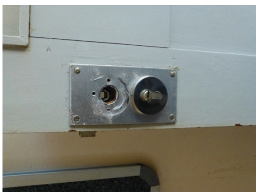
Photo 11: Broken doorknob (Chissano school)
