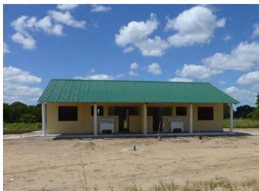
Photo 6: Teachers' house of Manjakaze school (under construction)
