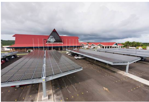
PV modules at the airport (on the roof of the parking lot) 「photo: JICA/Kaku Suzuki」
