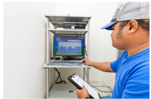
Power generation data is collected during the daily inspection 「photo: JICA/Kaku Suzuki」
