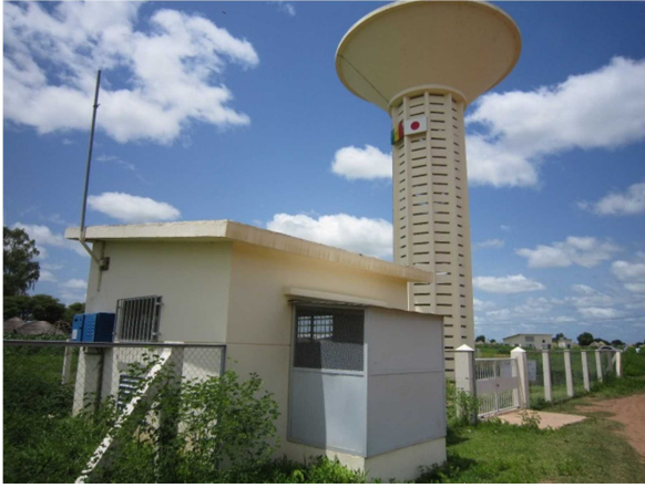
One of the renovated water supply facilities in the target sites, Sinthiou Maleme
