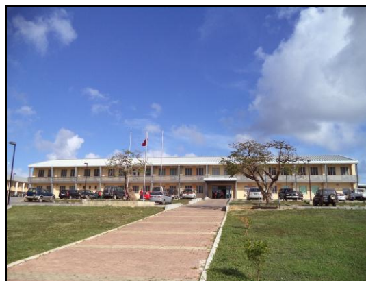
Outpatient Department Building Constructed in the Project
