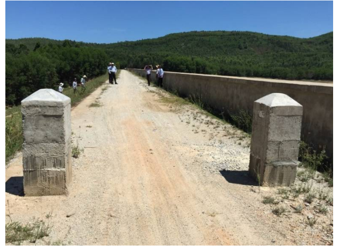
(Concrete poles for preventing trespassing of big trucks into An Tho reservoir site)
