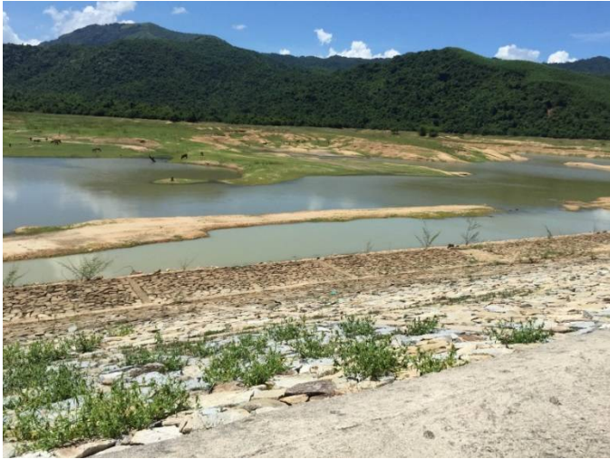
(Upstream of the dam body of Huan Phong reservoir)
