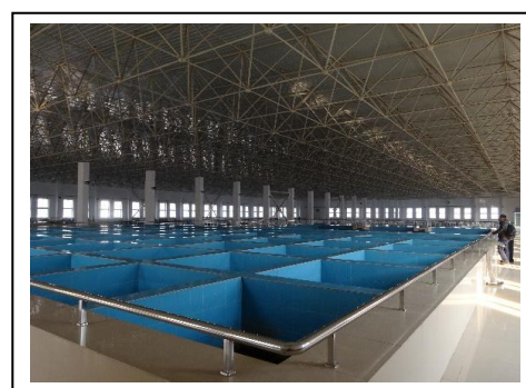
Photo1: A Purification Plant Built with This Project
