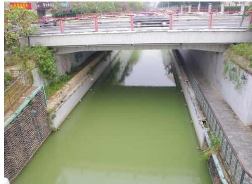
Photo 9: Discharge to the Yongjian River
