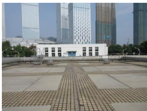
Photo 4: The biological reaction pool of the Treatment Plant
