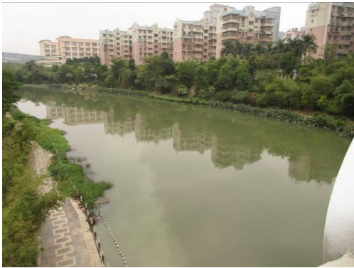
Photo 2: A revetment built on the Zhupaichong Stream
