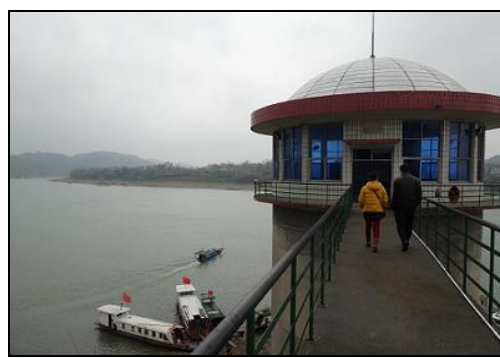
After the project, water is pumped up from the river, and sent to each household after being purified in the plant
