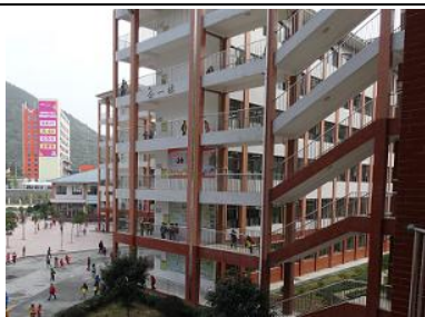
Education Subproject: Jishou City No. 8 Elementary School
