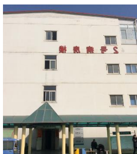
An infectious-disease ward. The building is designed to control infection through the use of design aspects such as negative pressure and double (isolated) corridors (Anyang).
