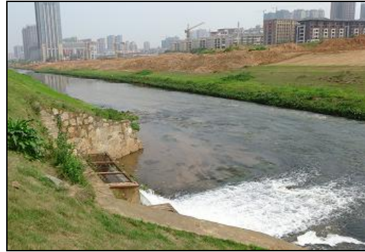
Photo 3: Guitang River into which the Xinkaipu Wastewater Treatment Plant discharges its treated water
