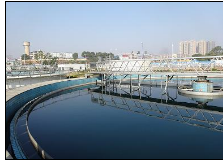
Photo 2: Liaojia Citang Water Purification Plant
