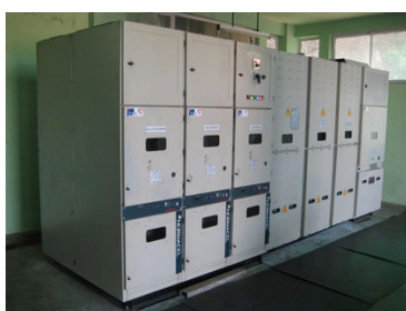
11KV Switch Gear Panel
