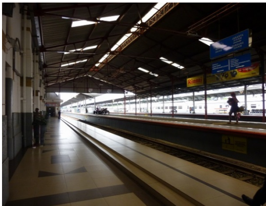
Photo 4: Inside the Kejaksaan Station after Rehabilitation
