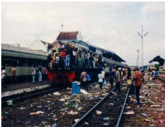
Photo 3: Kejaksaan Station before Rehabilitation (safety issues were prominent: the platform was low and people would enter inside the track to sell various things.)
