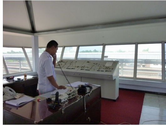
Photo 8: Developed Control Tower and Operation Control Device
