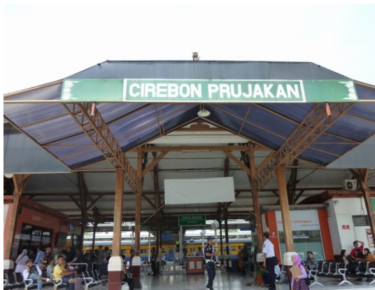
Photo 1: Rehabilitated Prujakan Station
