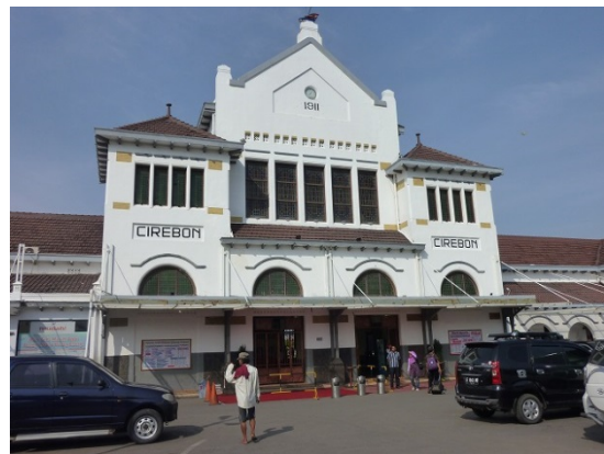
Photo 2: Rehabilitated Kejaksan Station
