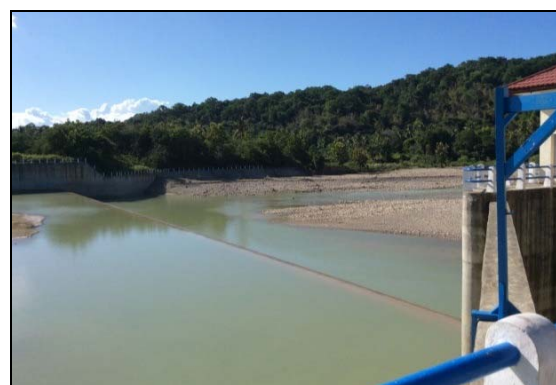
Constructed Weir of Malaka Weir Irrigation Project
