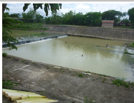
Revetment and riverbed repaired by the project (O&M agencies and residents remarked, “river flow became smooth”, etc.)
