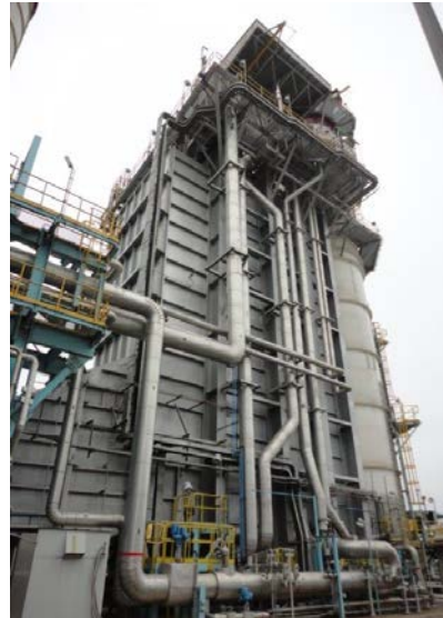
Heat Recovery Steam Generator
