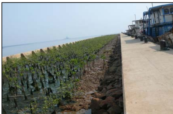
Photo 9: Breakwater using Mangrove (2011) Source: DGCF
