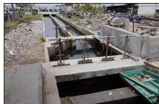
Photo 8: Sea Water Cleaning System (At the time of the Ex-post Evaluation)
