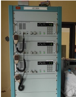
GMDSS (VHS/DSC) Equipment (Kalianget CRS)
