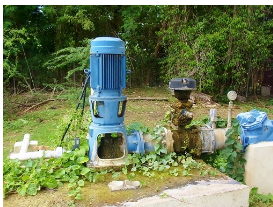
A well without proper cleaning (Cookson 3 Well)
