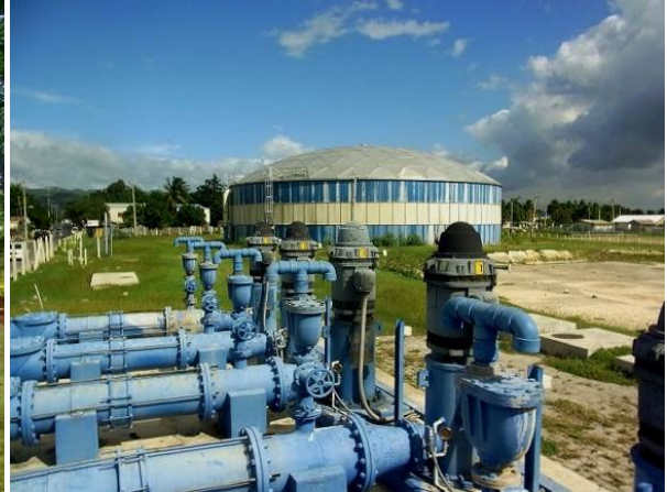
Reservoir and Distribution Pumps next to the WTP
