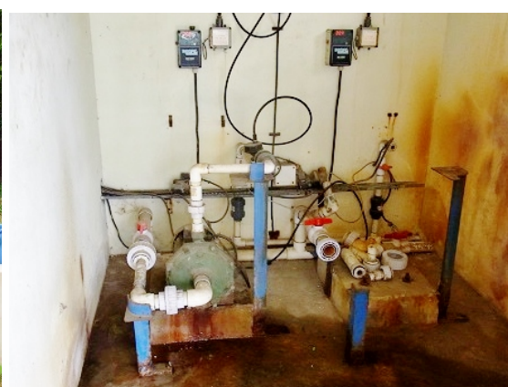
A well for which one of the chlorine injection pumps was removed to take spare parts (Friendship Well)
