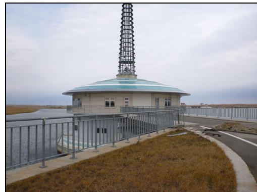
Water Intake Facility Constructed by the Project
