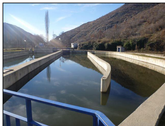
Photo 2: Water Intake No.3
