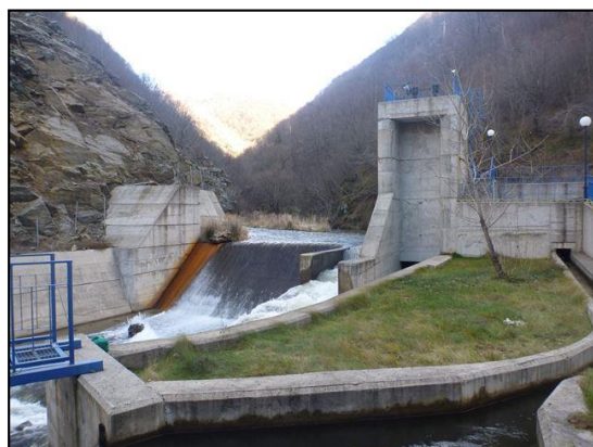
Photo 1: Water Intake No.1
