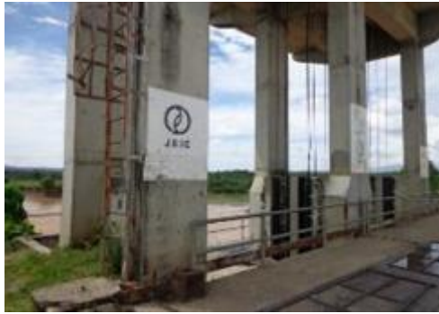
Photo 3: Sluice Gate (double lift) [at the ex-post evaluation]
