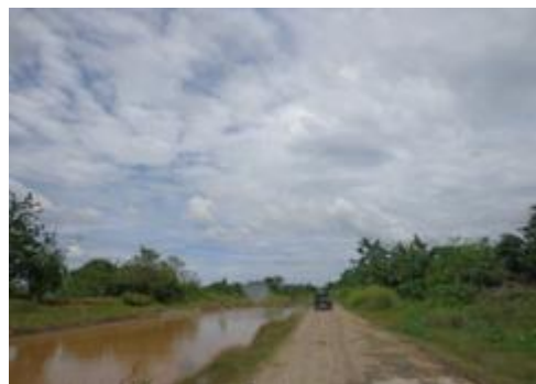
Photo 2: Diversion Canal leading to the Diversion Dam [at the ex-post evaluation]
