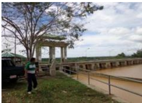
Photo 1: Maridagao Diversion Dam [at the ex-post evaluation]
