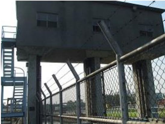
Flood gate of a pumping station constructed by the project
