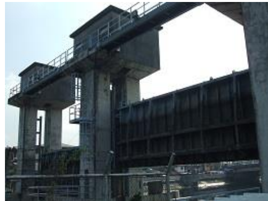
Flood gate constructed by the project
