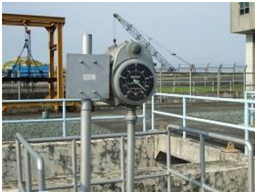
Pumping station constructed by the project
