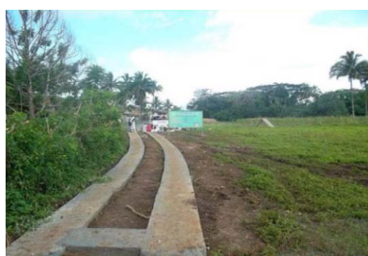
Concrete Tire Path Tubaran, Lanao del Sur
