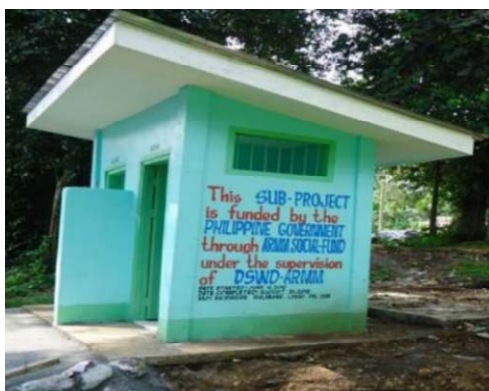
Water and Sanitation Facilities Malabang, Lanao del Sur
