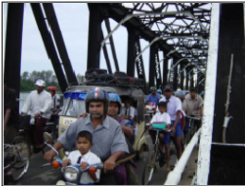
Congestion at Kallady Bridge Before project
