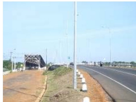
Kallady Bridge (Left bridge is an old bridge) (Picture provided by Oriental Consultants Co., LTD)
