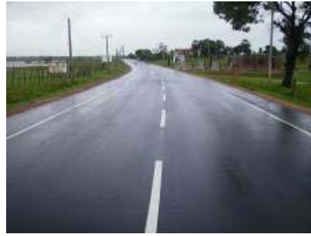
National Road A15 at Trikkandimadu After project
