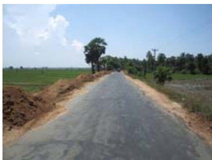
National Road A4 at Addalachchena Before project
