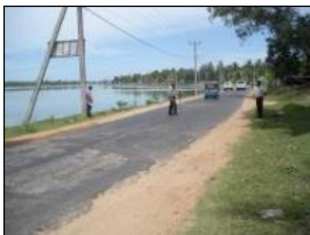
National Road A15 in Batticaloa Before project
