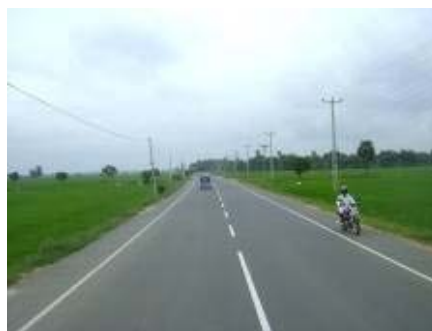
National Road A4 at Addalachchena After project
