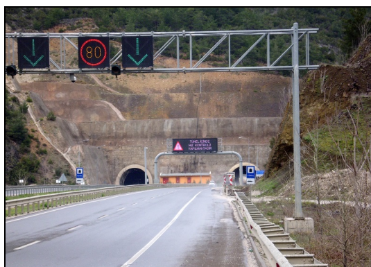
Photo 1: Tunnel of the State Road D650
