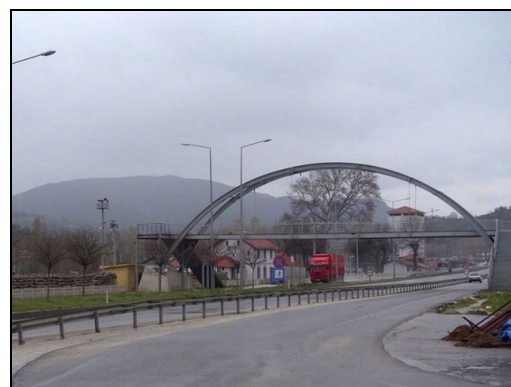
Photo 4: Pedestrian overpass on the State Road D650
