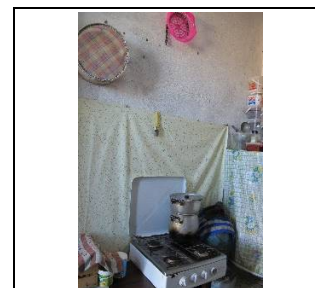
A fluorescent light is installed in the kitchen of an SHS-installed home in Tataouine
