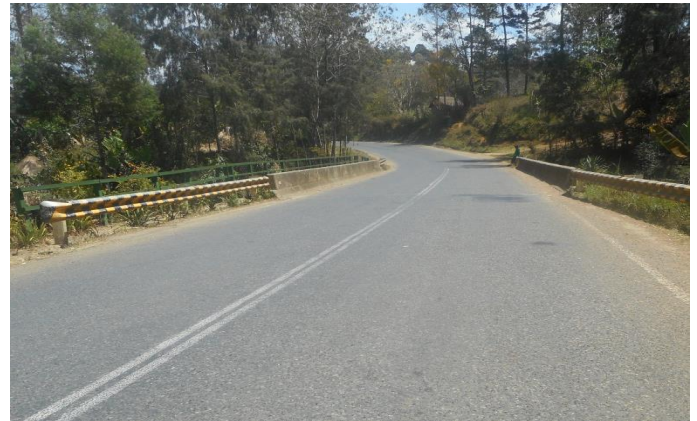
Orompaka bridge with two-track
