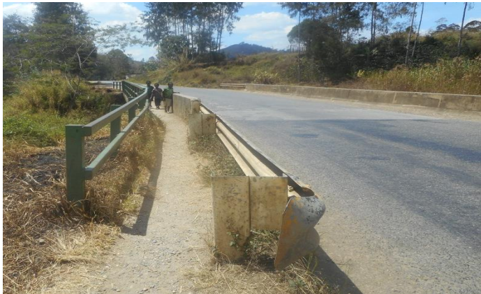
Ofiga bridge with hand rail and walk way
