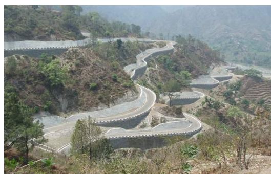
Road Improved by this Project 2
