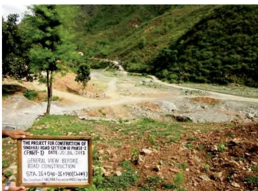
Photograph 1: Before the Construction 16
