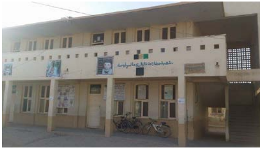
School Building Abdula Ahad Karzai Middle School (Kandahar City)
