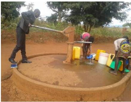
Water supply facility provided by the Japanese grant aid project in Vacha Community, Alto Molocue
